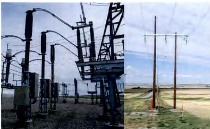
*Left: A typical 240kV circuit breaker*
